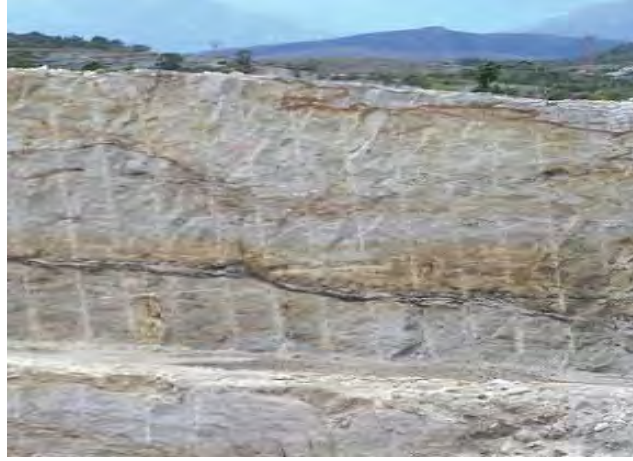
Figure 2. Hole paths left by presplitting
