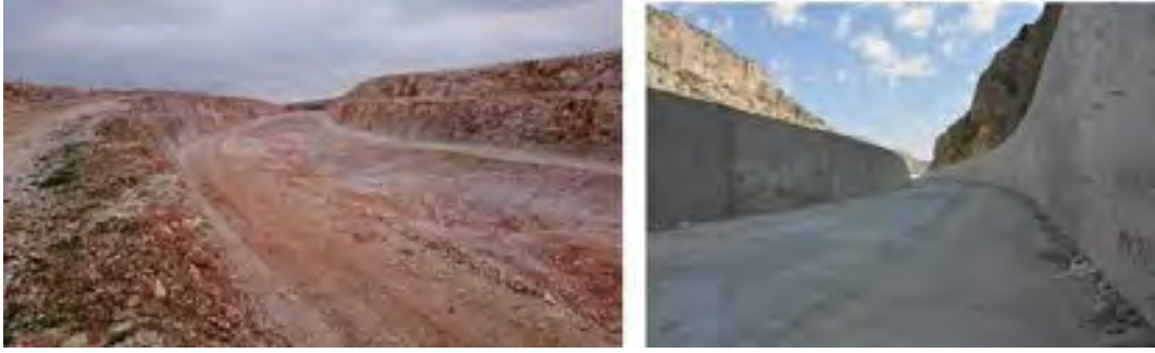
Figure 7. Irrigation channel section
