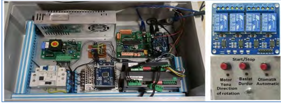
Figure 5. Control unit, 4-channel relay card, and manual usage unit
