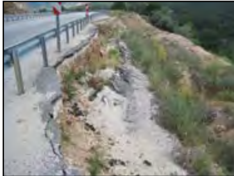
Figure 4. The Landslide and the deformations
