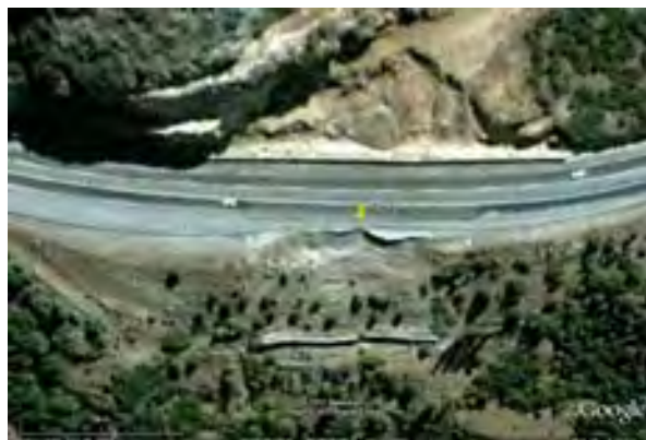
Figure 6.The satellite photo of the landslide in 2003.
