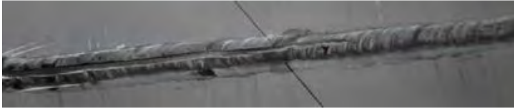
Figure 5. Welded zone and damage that applied of it surface.
