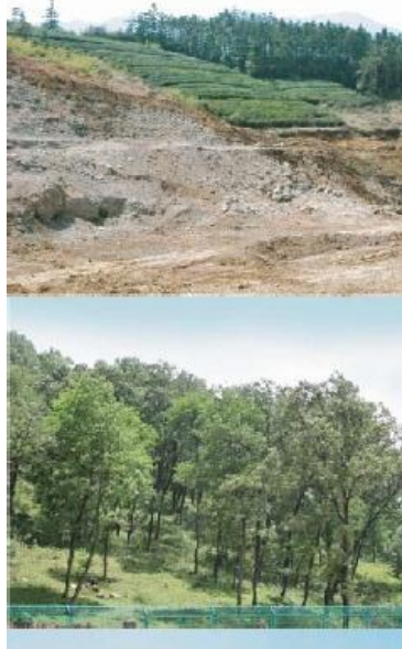
Figure 5: Before and after photograph in construction site of roadway
