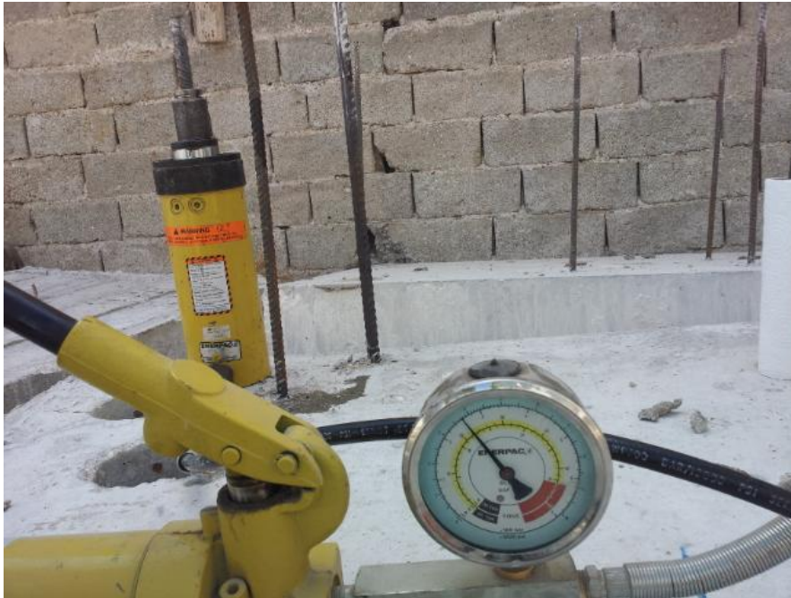
Fig.3. Hydraulic test apparatus of anchor rebar.
