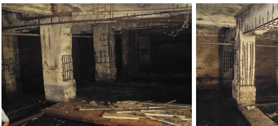
Figure 3. The groundwater and the situation of load-bearing members in the foundation level
