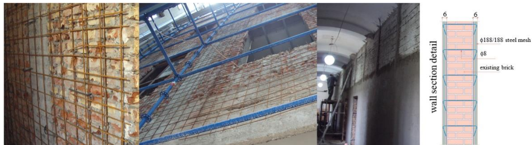
Figure 9. The using of the steel meshing in the wall strengthening
