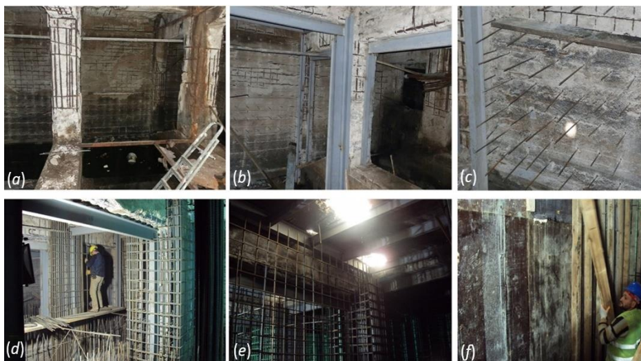
Figure 7. Strengthening applications on the basement floor: (a) The drainage of the existing water, (b) The application of the steel profile columns and beams, (c) The anchor holes in the existing RC system and the connections of the rods via epoxy, (d) The connections of the steel bar in the foundation, columns and beams, (e) The connections of the shear walls between the columns, (f) The building-up the wooden formworks and the construction of the self-compacting concrete.
