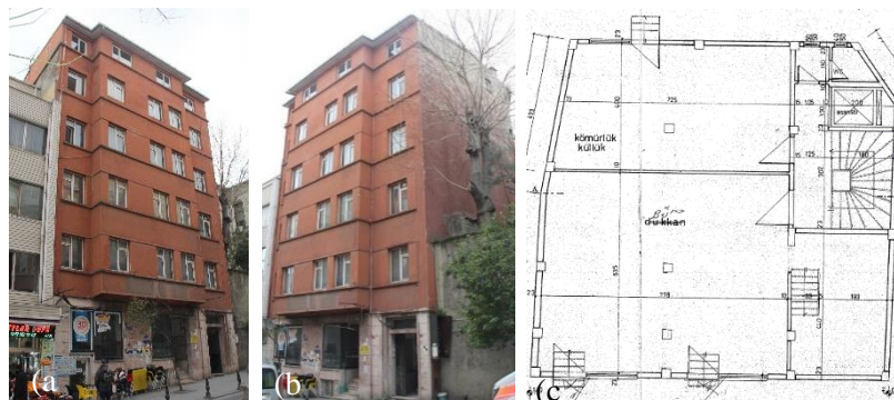
Figure 1. General overview (a,b) and layout (c) of the investigated building
