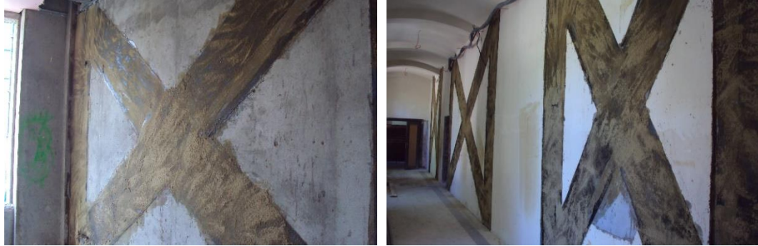
Figure 10. The using of carbon fiber in the wall strengthening
