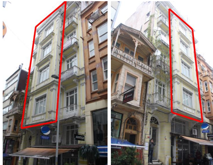
Figure 3. Investigated frontal facade wall of the building
