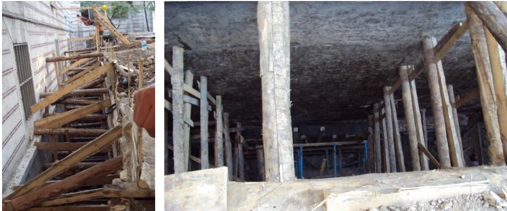
Figure 5. Well foundation construction (Excavation works at -12.80 m.)
