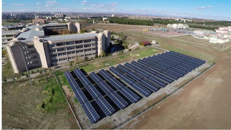
Figure 6. View of solar energy panels at Dicle University.
