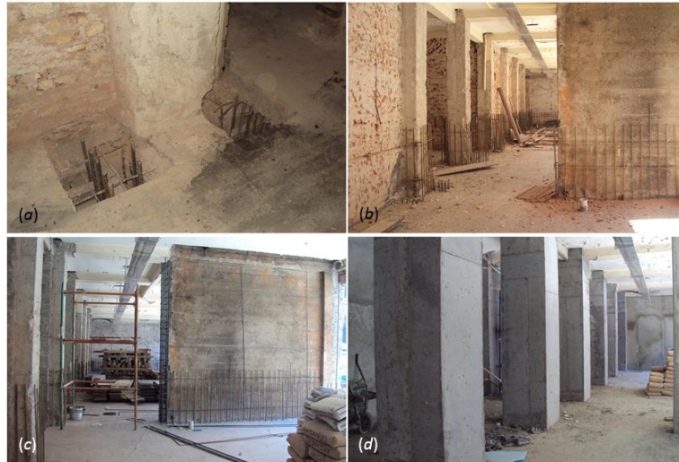
Figure 8. Jacketing application process on the ground floor (a-d)
