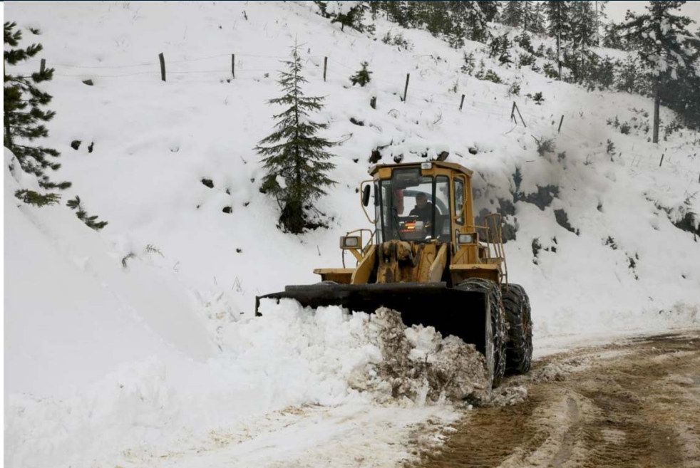
Figure 3. Dozer Cleans the Roads
