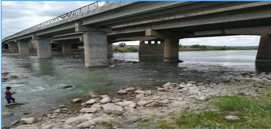
Figure 3. Bottom view of Sadi Bridge
