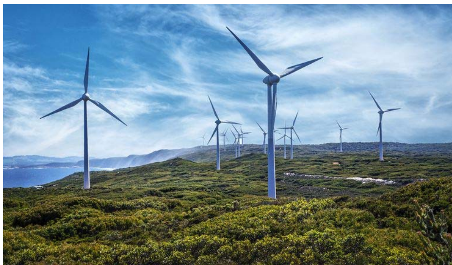
Figure 2. On-shore wind power plants
