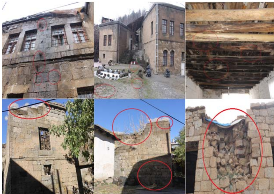
Figure 4. Observed Damage Historic in Bitlis Houses
