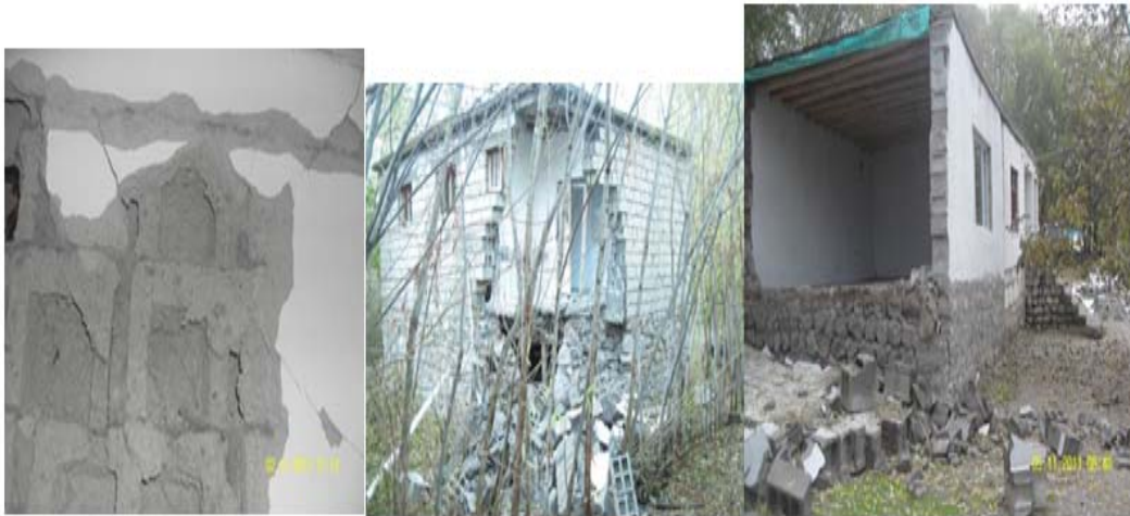
Figure 2. The damages of concrete briquette walls [5,6]
