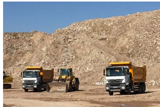
(b) Equipment in the plant in Eskisehir
