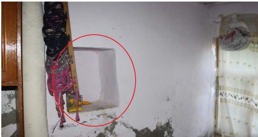
Figure 3. The Part Used as a Storage Area on the Inner Walls of the Historic Bitlis Houses
