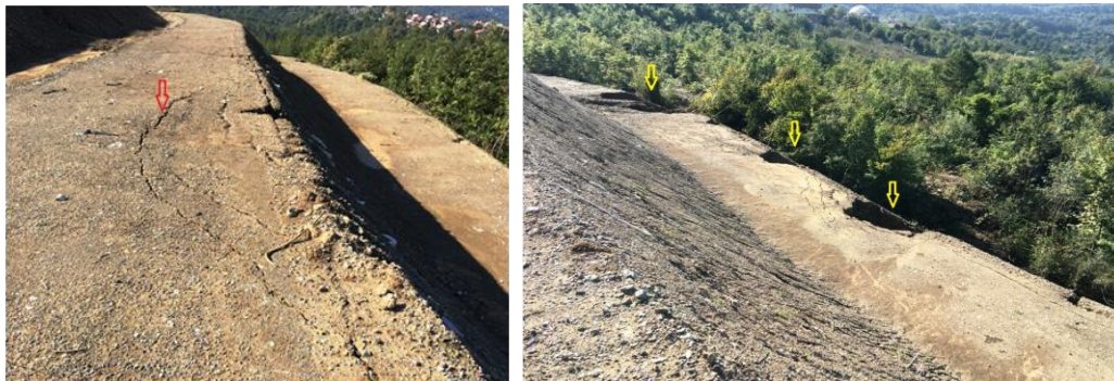
Figure 2. (a) Tension cracks appeared on the steps (b) Slippings existed at the steps
