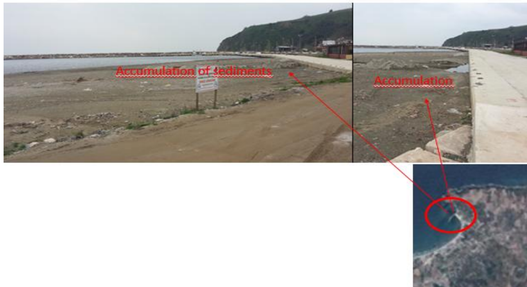
Figure 6. Outlook of a fishing harbor on Eskel beach area filled with sediments
