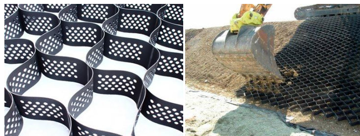
Figure 16. Slope surface protection with geocell material
