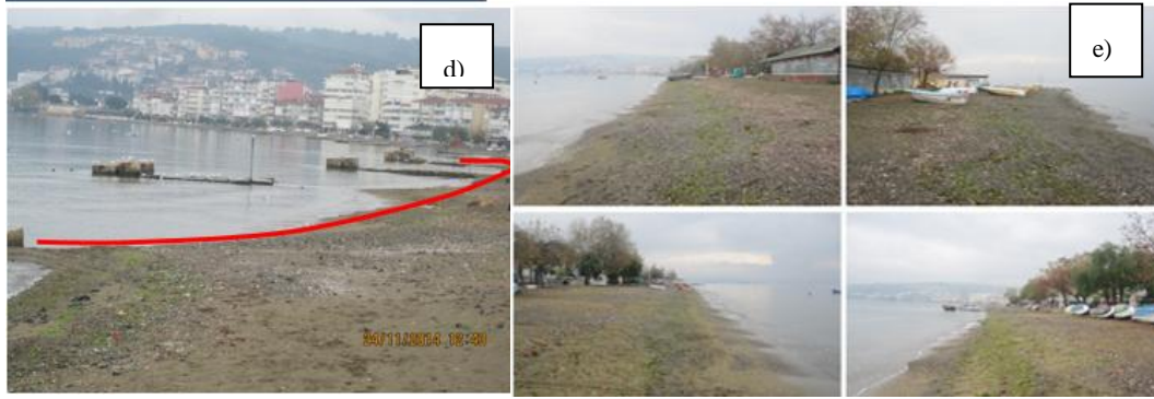
Figure 7. Outlook of Buyukkumla region and Kucukkumla beach, the region with groins and no groin and with accumulation and erosion
