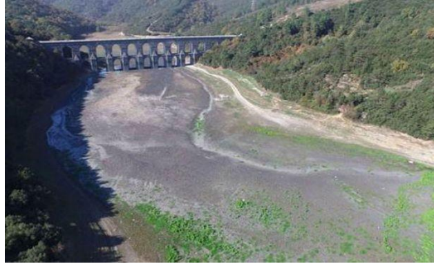
Figure 1. The view of the unloaded dam.
