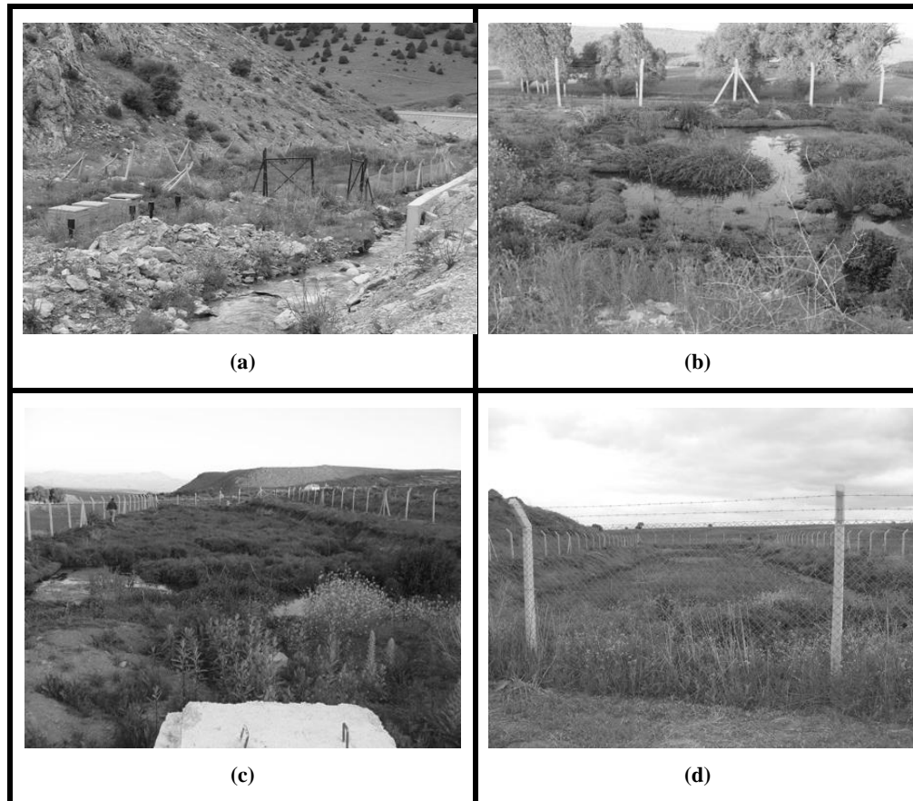
Figure 5. Common failures experienced in practice (Gokalp et al., 2014)
