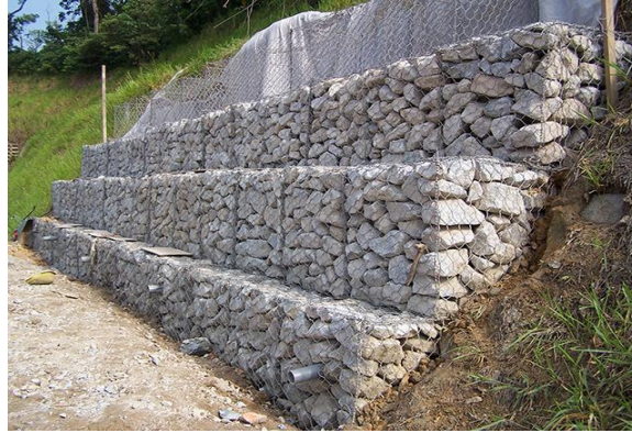
Figure 12. Gabion application with rock filler
