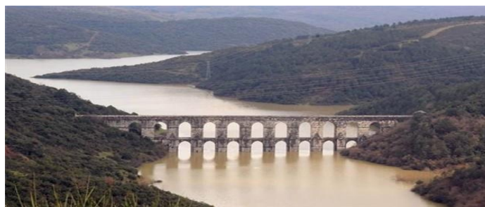
Figure 2. The view of the loaded dam.
