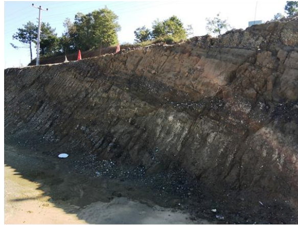
Figure 1. A view of a section of the natural soil stratum
