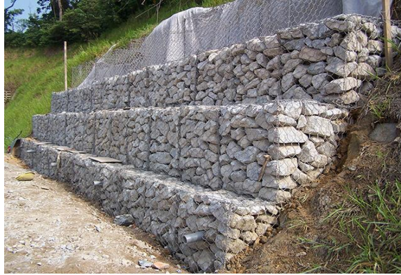
Figure 12. Gabion application with rock filler
