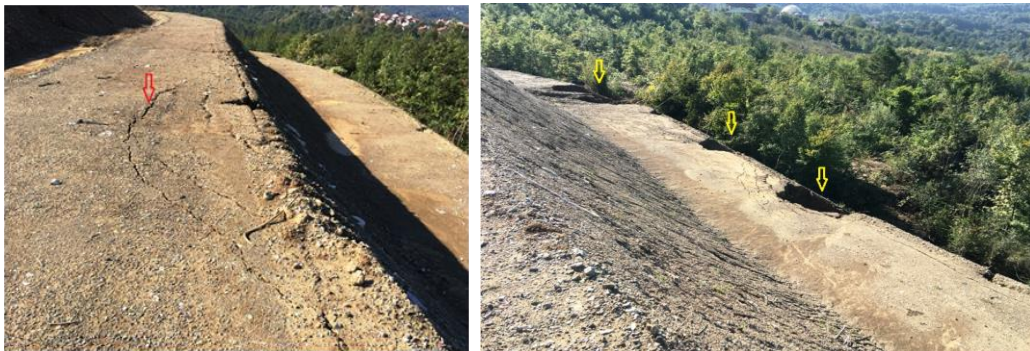
Figure 2. (a) Tension cracks appeared on the steps (b) Slippings existed at the steps
