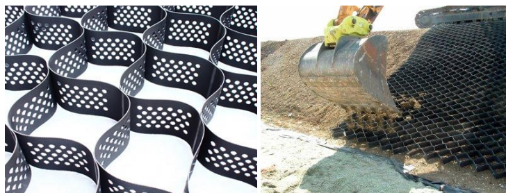
Figure 16. Slope surface protection with geocell material
