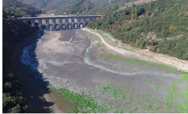
Figure 1. The view of the unloaded dam.
