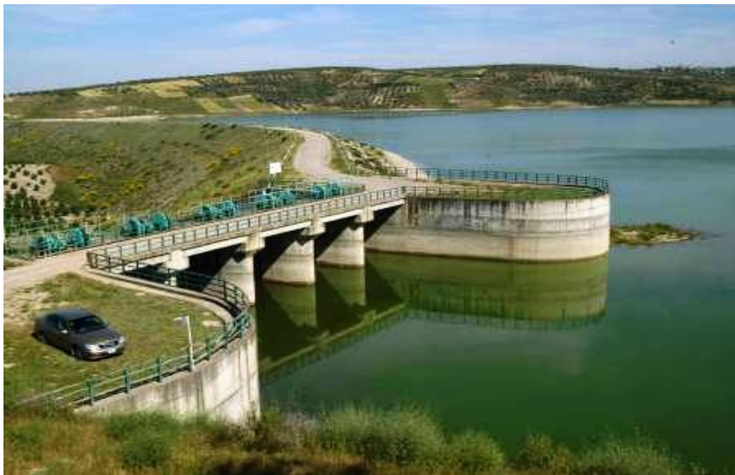
Fig.2 General view of Yarseli dam
