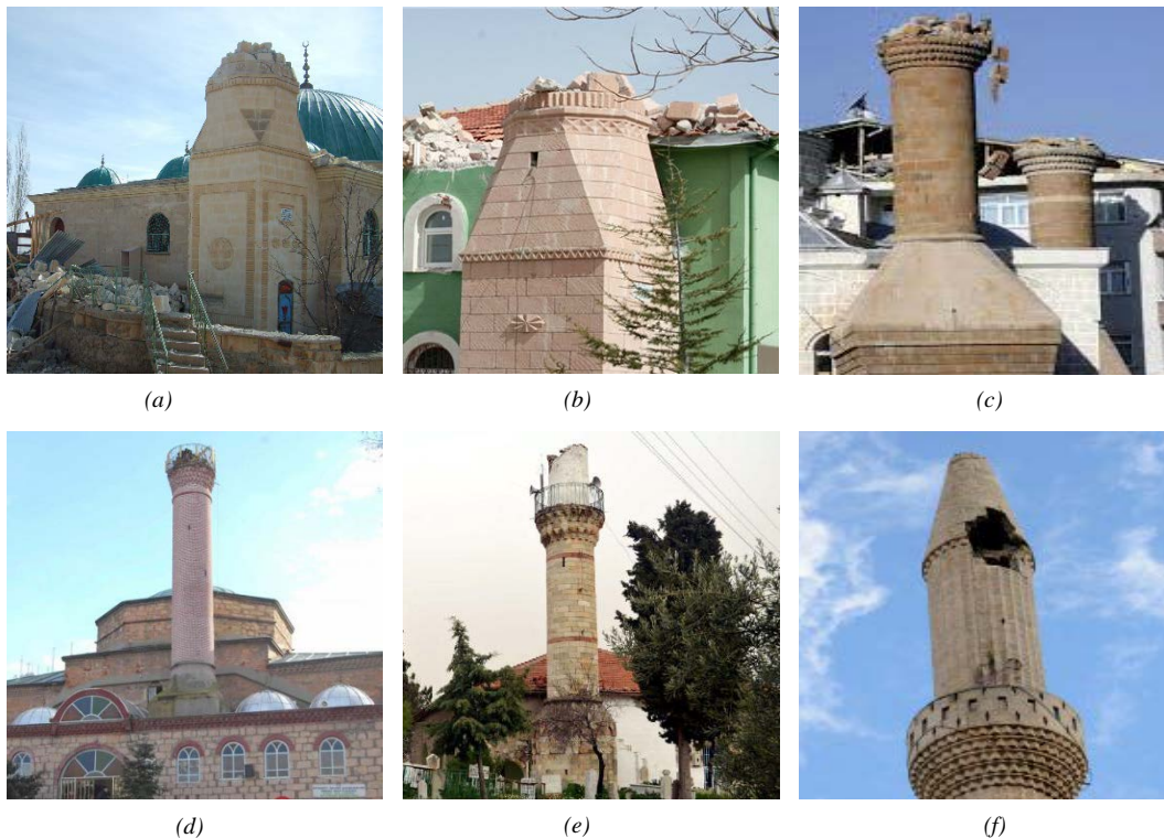
Figure 7. (a) Collapsed minaret due to the storm, Konya/Bozkır, 2010, [7] (b) Collapsed minaret of Elmacık Mosque due to the storm, Elmacık/Aksaray, 2013, [8] (c) Damaged minarets of Van Yolu Mosque due to the earthquake, Erciş/Van, 2011, [9] (d) Damaged minaret of Nasuh Ağa Mosque due to the earthquake, Simav/Kütahya, 2009, [10] (e) Damaged minaret of Balaban Paşa Mosque due to the storm, Aliağa/Izmir, 2015, [11] (f) Damaged minaret of Yavuz Sultan Selim Mosque due to the thunderbolt, Kilis, 2016, [12]
