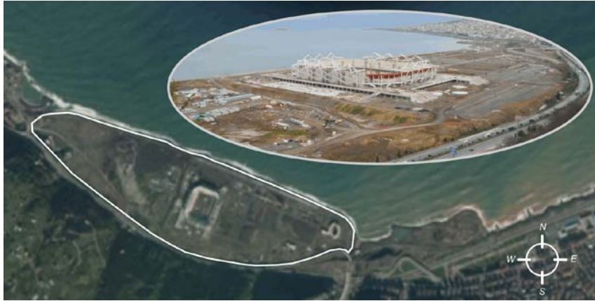
Figure 1. Gross construction area of the Akyazı Spor Complex and the Akyazı Stadium viewing [4;5]
