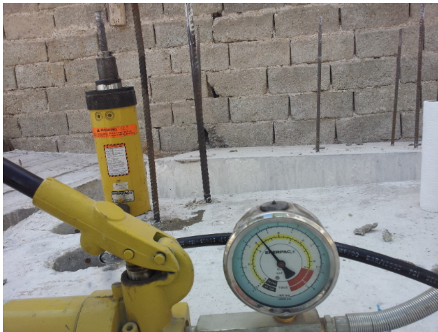
Figure 3. Hydraulic test apparatus of anchor rebar.
