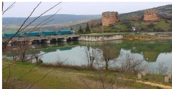
Figure 2: Aerial view of the dam
